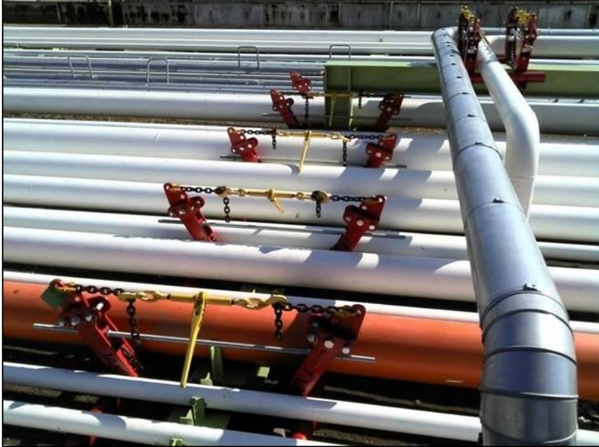
An example of 5 tools lifting a total of 16 pipes in unison.
