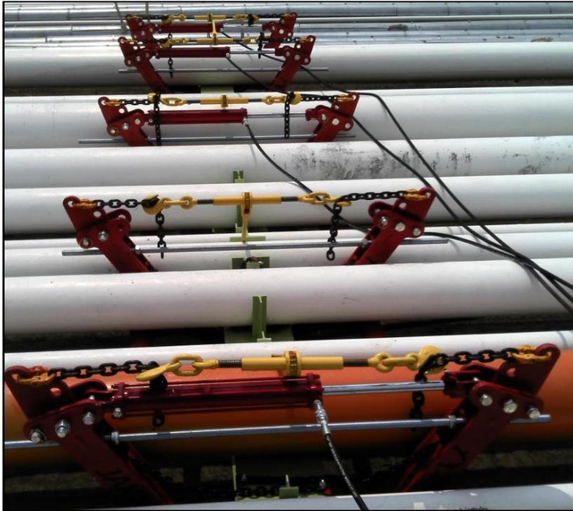
Initial lifts (break-aways) are done remotely using hydraulic activation to avoid personnel exposure if there is a loss of containment at suspect contact areas. This enables our ability to conduct in-service remediations.
